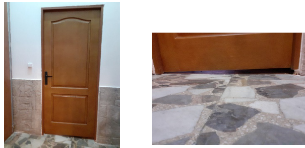
Fig 10. The warehouse entrance door
